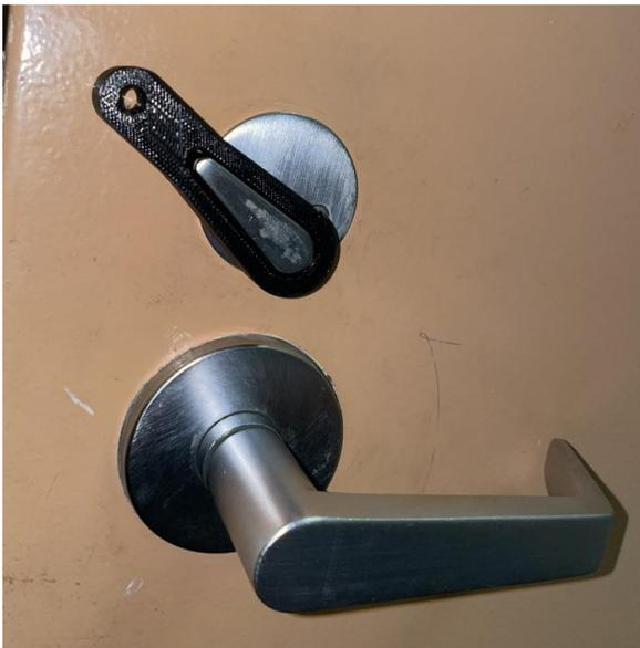
Figure 10: Door lock fitting placed on the door lock
